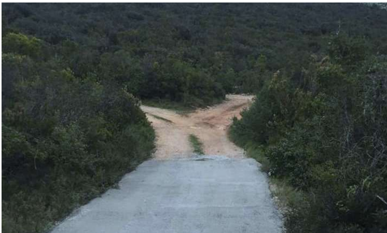
Betoniranje puteva u krajoliku https://www.facebook.com/MO-%C5%BDrnovo-Postrana
